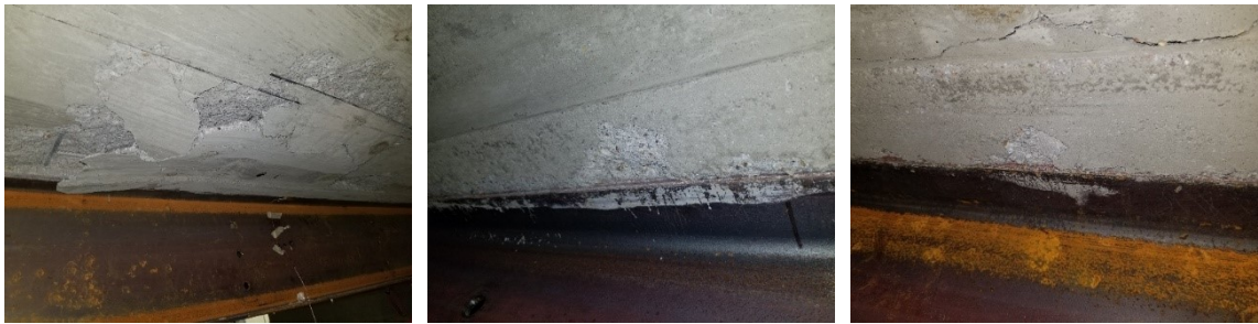
(a) Interior stringer near Loc. 3 (b) Exterior stringers near Locs. 13 & 17 (c) Interior stringer near Loc. 10
