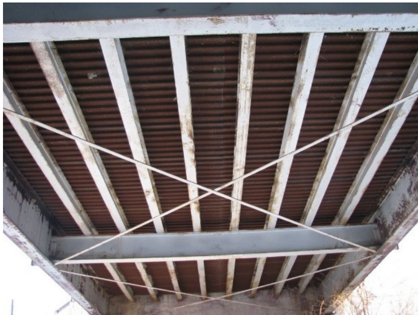
Figure 1. Sample floor system, fascia girder
